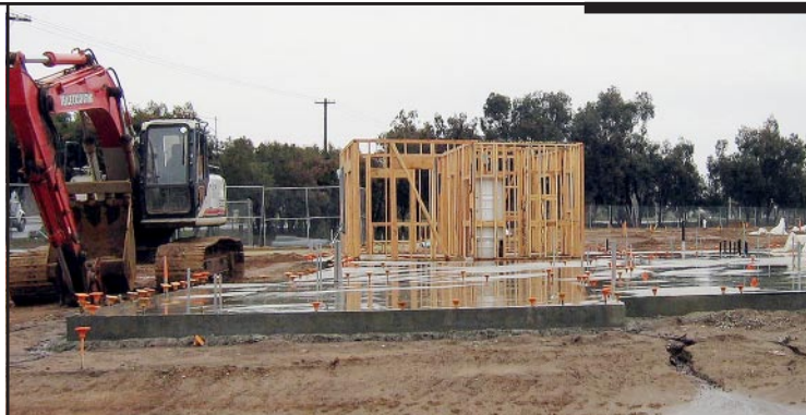
MLK VILLAGE CONSTRUCTION
